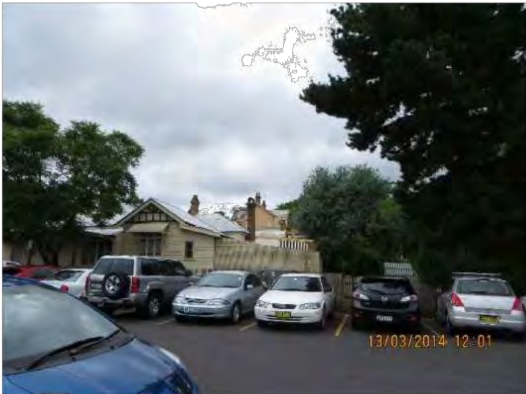
Figure A-29: Proximity to Adjoining Properties
